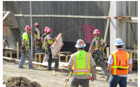
Coordinated effort to install noise wall panels along eastbound US 36
